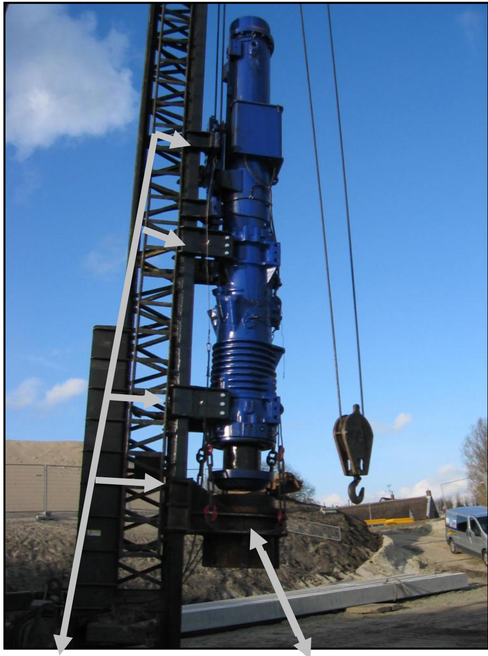
Guiding for starter , diesel hammer and pile cap.
